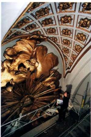
Fig. 6: Condition survey by mapping of the stucco altar in Maria Magdalena church. Photo: H.
