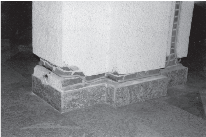
Fig 8a u. b: The Sacro Cuore Church. Installation of the tempering system. There was no need to preserve the original plaster. Photos Thomas Becker, Milan.
