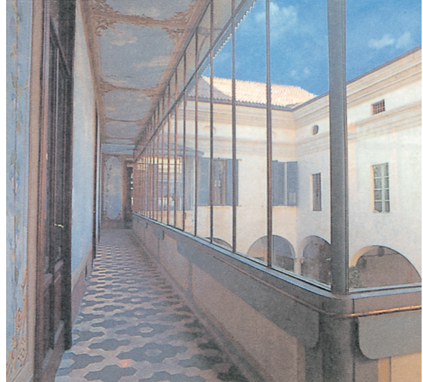
Fig. 4: Palazzo Cattaneo, Ala Ponzone. Pompeian Gallery. The water and electrical lines are mounted on the building elements: The two heating pipes are under a layer of mortar at the base of the outer walls. On the floor in front of these, underneath a hollow molding, are the electrical cables, which also supply the lighting fixtures mounted on the wall. Photo Alberto Grimoldi, Milan.
