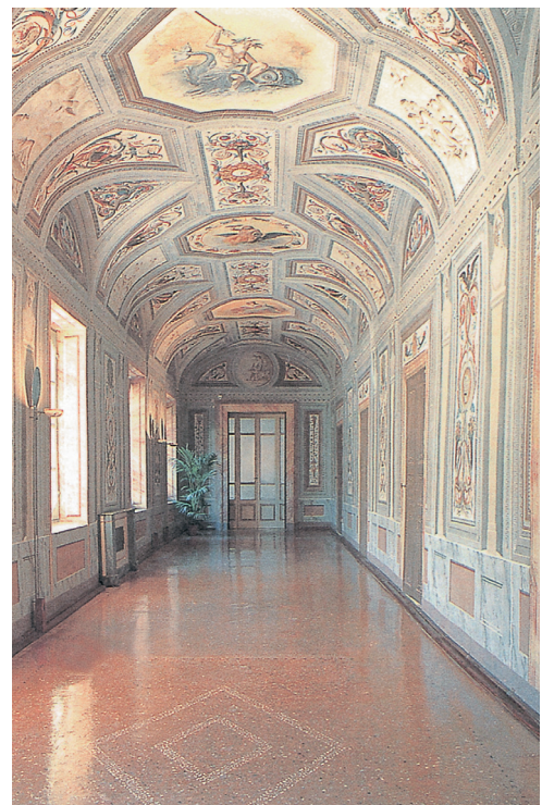
Fig. 4: Palazzo Cattaneo, Ala Ponzone. Pompeian Gallery. The water and electrical lines are mounted on the building elements: The two heating pipes are under a layer of mortar at the base of the outer walls. On the floor in front of these, underneath a hollow molding, are the electrical cables, which also supply the lighting fixtures mounted on the wall. Photo Alberto Grimoldi, Milan.
